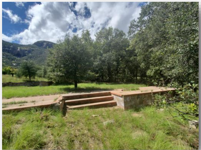
Foundation of the Healy's Ranch home.
